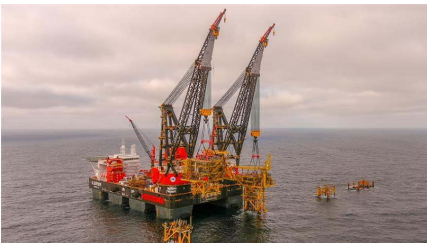
Figuur 5-9: Topside installatie met de Sleipnir ( https://www.energyfacts.eu/totals-tyra-production-topside-installation-successfully-completed/ )
