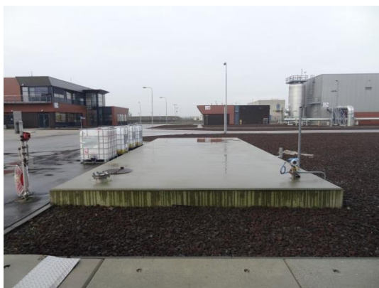
foto 1: Open drains tank
