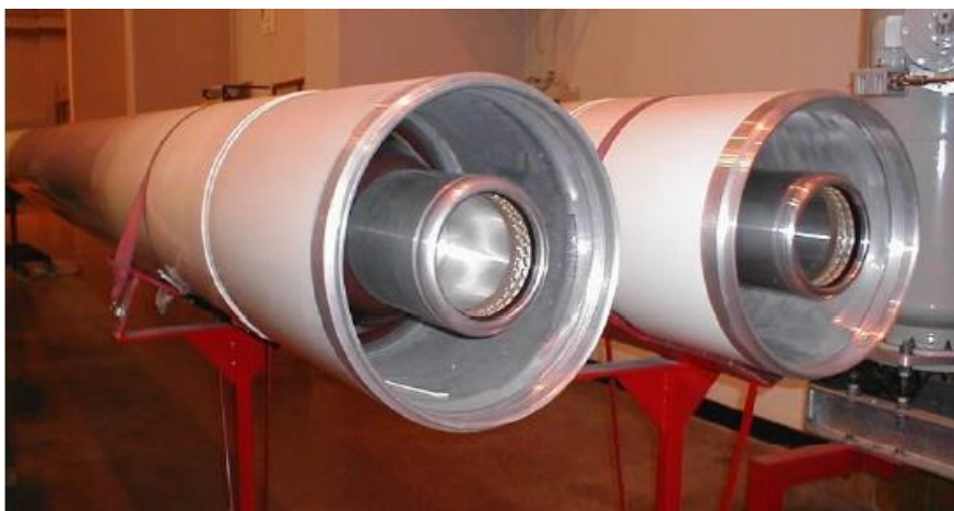
Figure 3 Gas insulated line construction details
