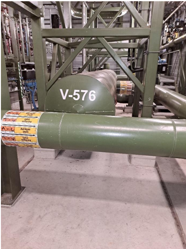
Objectnr. 78 V-576 Acoustical discharge filter
