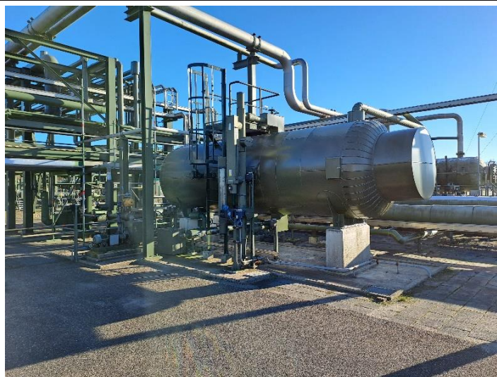
Objectnr. 51 V-020 Flare drain vessel
