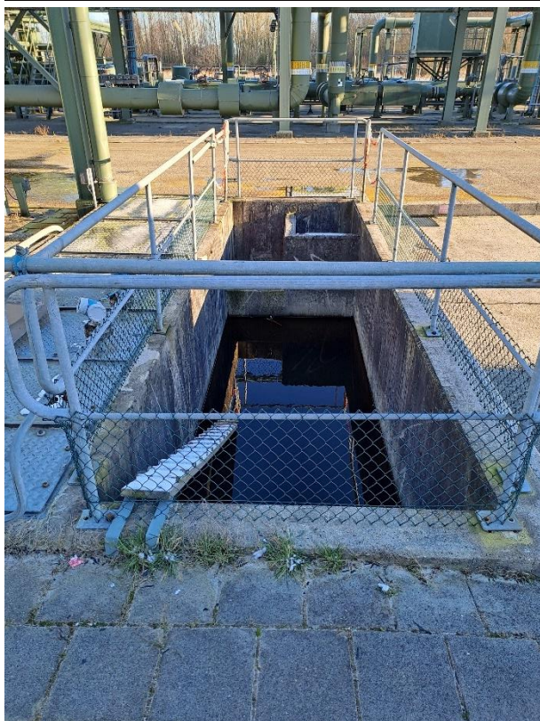
Objectnr. 36 V-082 Slug catcher drainpit
