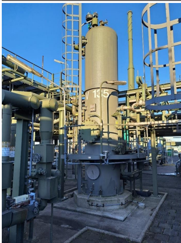
Objectnr. 11 V-135 Buffer vessel
