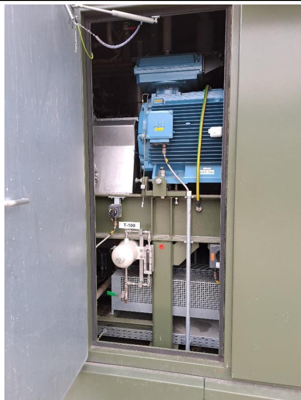
Objectnr. 81 K-100 HC-gas screw compressor
