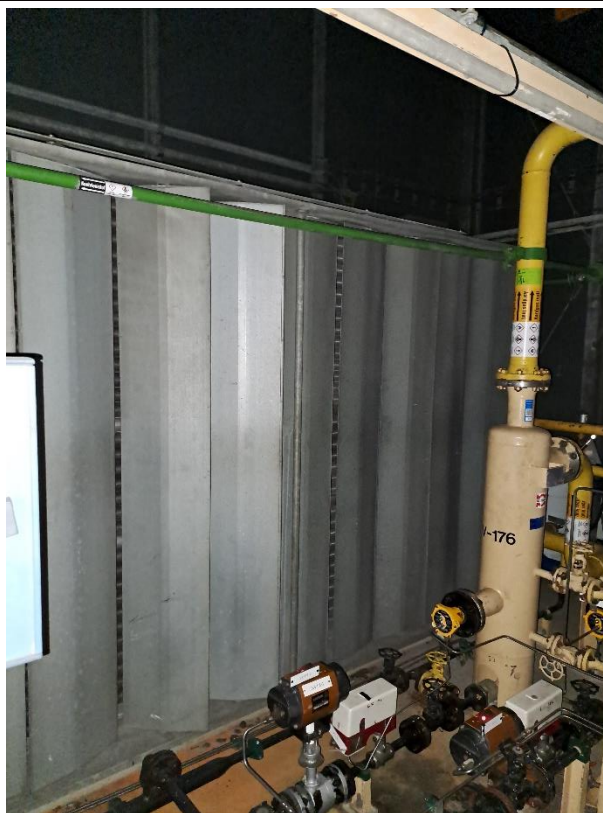
Objectnr. 21 E-179 2nd stage discharge cooler
