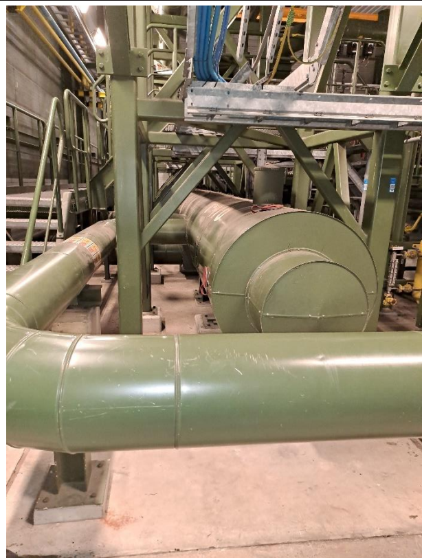
Objectnr. 73 V-476 Acoustical discharge filter
