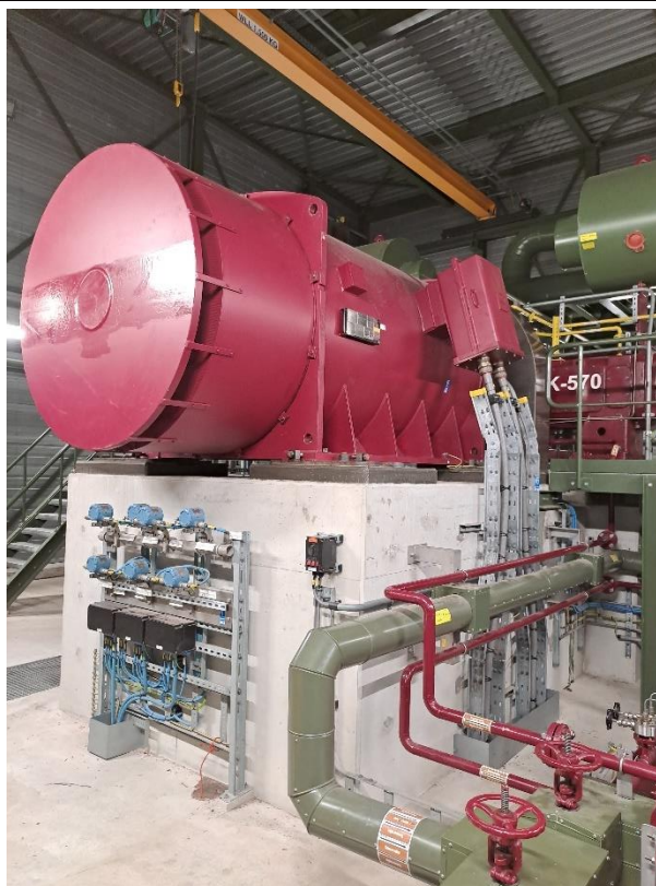
Objectnr. 75 K-570 HC gas compressor
