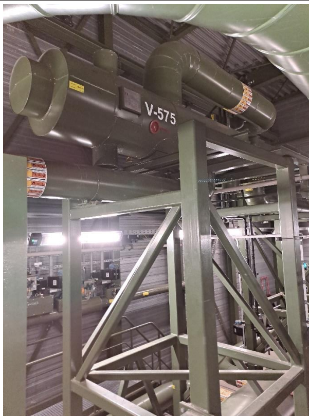
Objectnr. 77 V-575 Acoustical suction filter
