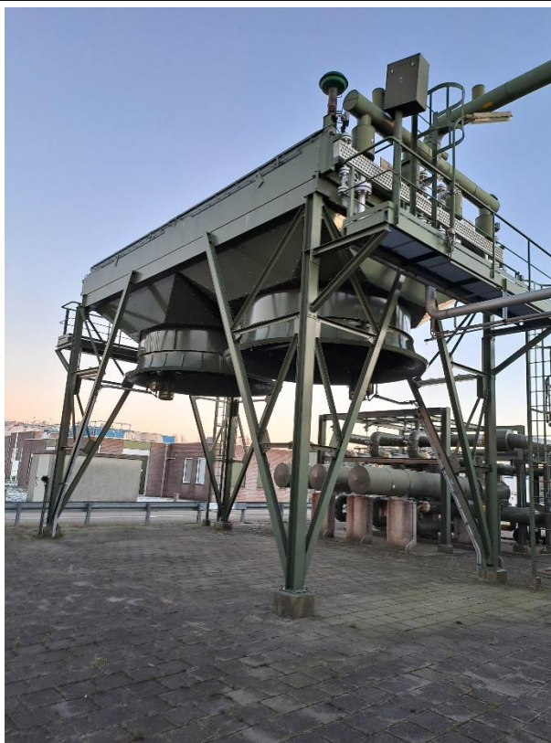
Objectnr. 17 E-123 Regenerator gas condensor
