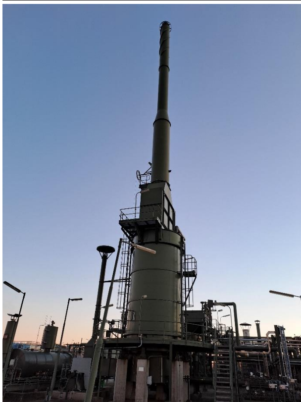
Objectnr. 22 F-122 regeneration furnace
