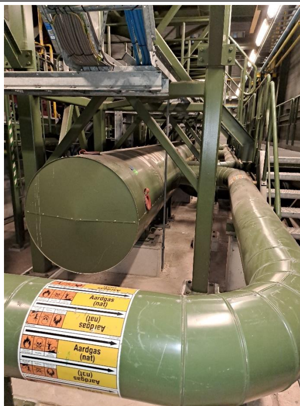
Objectnr. 67 V-376 Acoustical discharge filter
